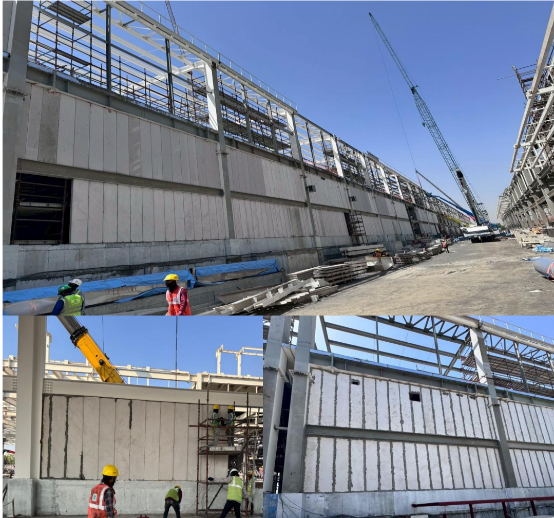
Industrial Project; Sanand
