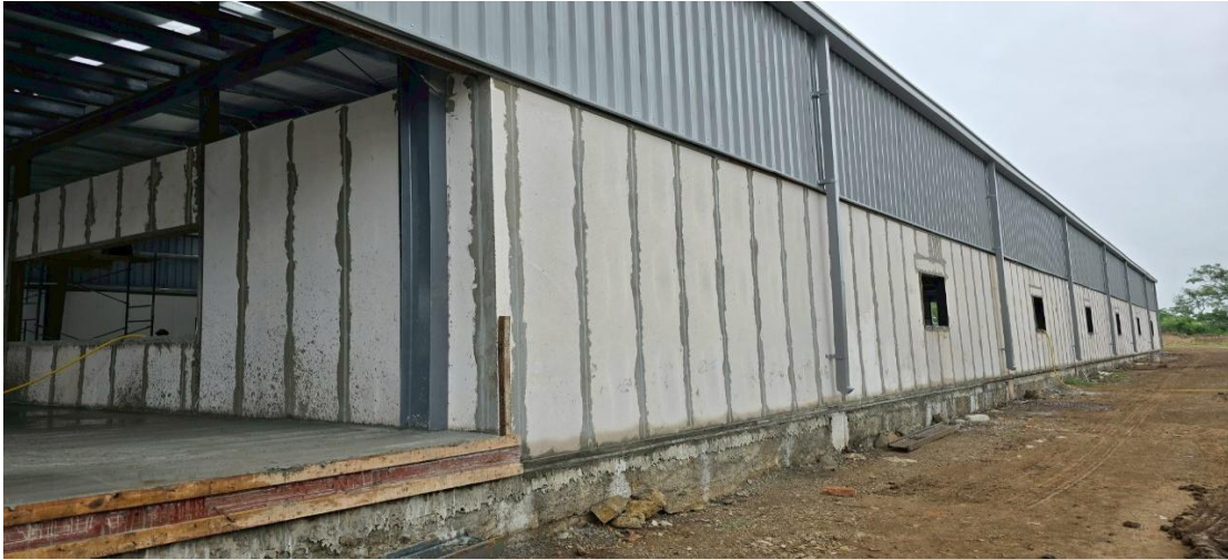
Car Showroom; Solapur
