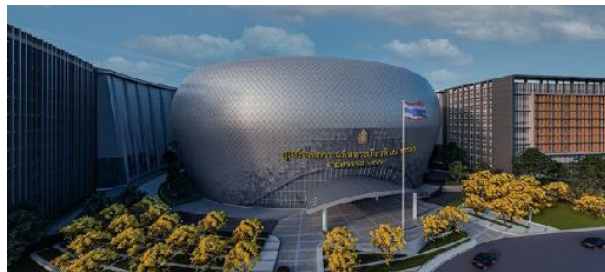
District Cooling System Thai Government Complex Center Zone C Bangkok, Thailand
