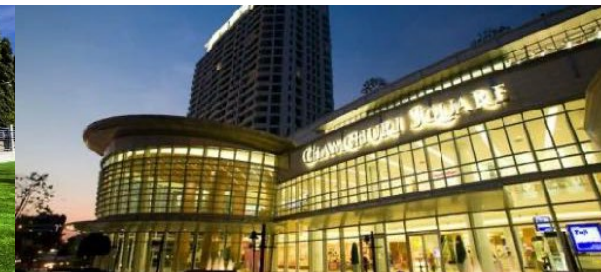
Chiller Plant Chamchuri Square, Bangkok, Thailand
